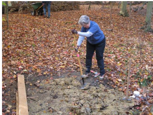
Figure 1. PVC pipe to control water levels was placed on degraded portion of trail and held in place with concrete prior to trail rehabilitation (left). Volunteer packing trail fill over water control pipe and adjacent to retaining wall (right).
