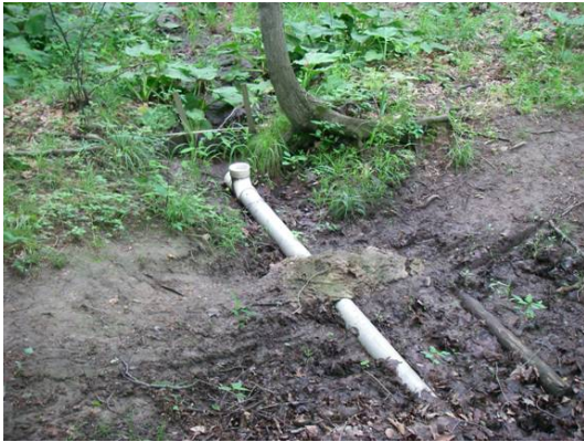
Figure 1. PVC pipe to control water levels was placed on degraded portion of trail and held in place with concrete prior to trail rehabilitation (left). Volunteer packing trail fill over water control pipe and adjacent to retaining wall (right).
